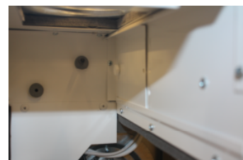
Picture 17: Summer bypass plate in the winter position.
