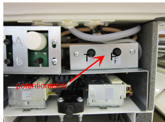
Picture 11: Location of the potentiometers(T=supply,P=exhaust).
