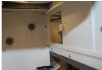
Picture 16: Summer bypass plate in the summer position.
