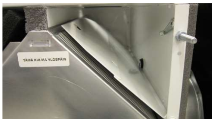
The heat recovery cell in the summer position, the bypass plate is turned in the front of the cell, the outdoor air passes behind the heat recovery cell.
