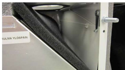
The heat recovery cell in the winter position
